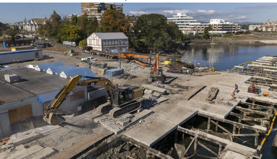
View of site demolition and machinery from over Inner Harbour.
