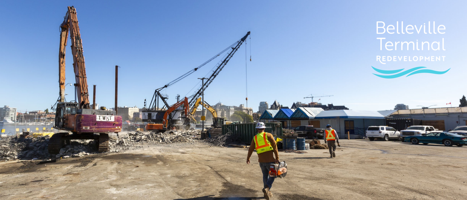
View of site demolition, machinery and workers.
