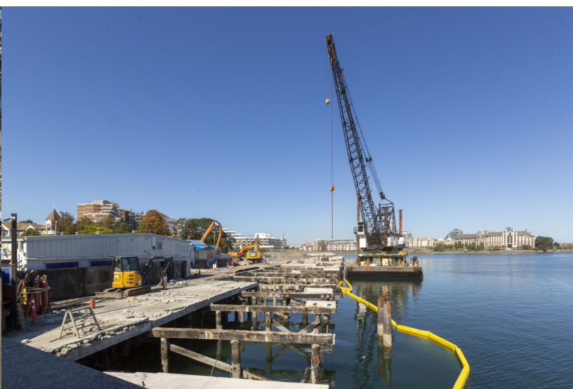
View of wharf demolition and barge crane from Inner Harbour.
