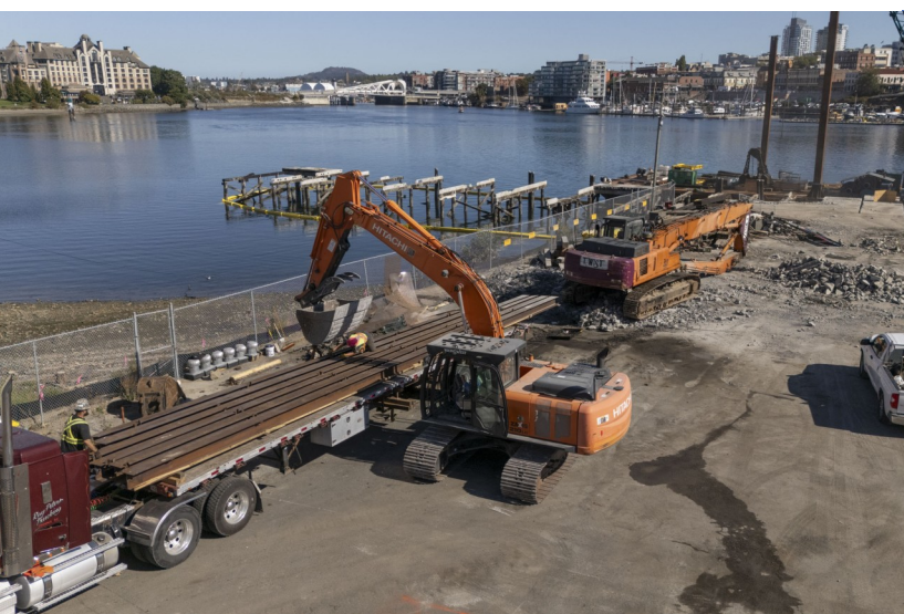
View of wharf demolition and machinery from site.
