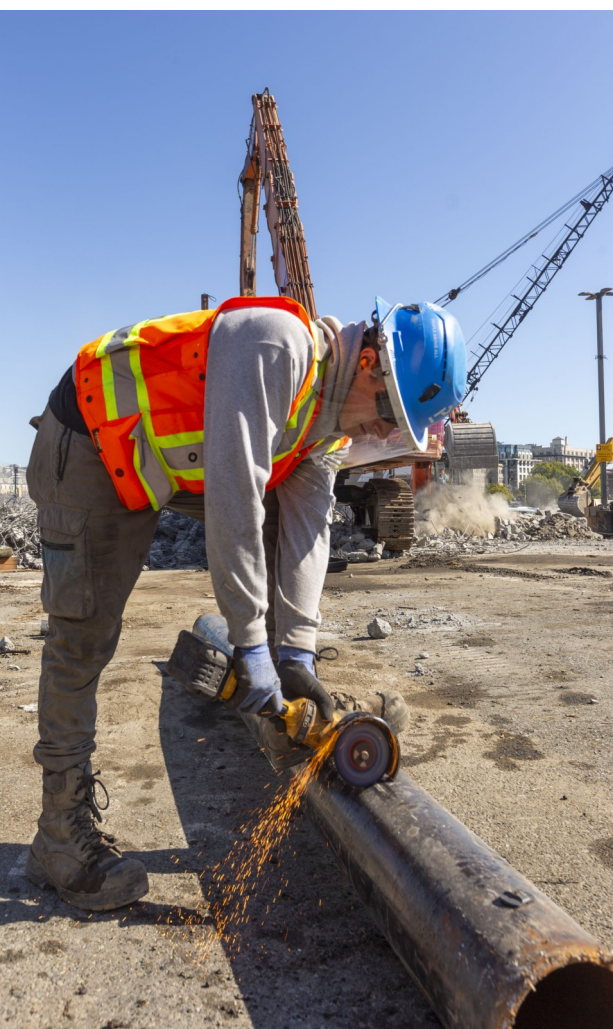
Site worker demolition.
