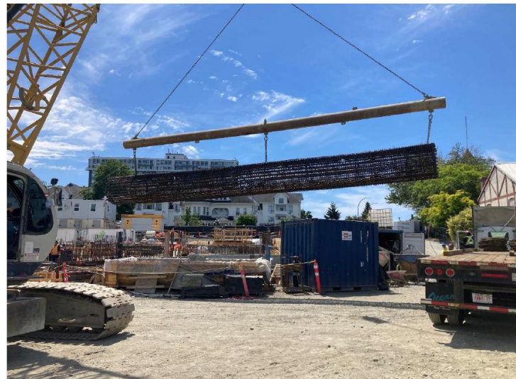
The crew unloads rebar cages. Photo taken June 2026.
