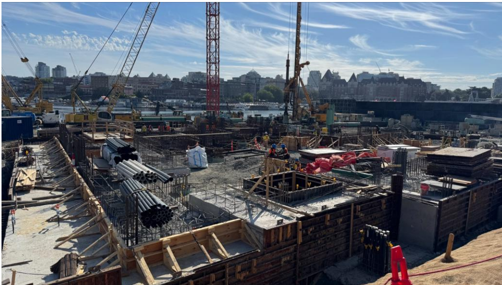
The site remains busy as crews build the foundation for the new terminal. Photo taken June 2026.
