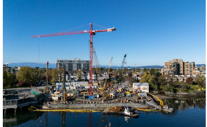
Figure 2: Aerial view of the site looking south showing a barge delivering construction supplies.
