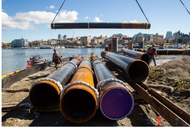
Figure 1: Piles for the retaining wall system are offloaded from a barge to site.
