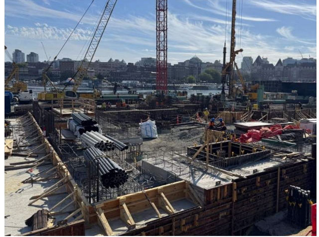
Figure 2: Progressing with building the foundation for the new terminal.
