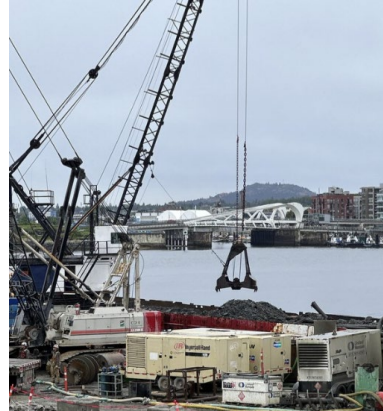
Figure 2: A crane loads material from dredging onto a barge for transportation from the harbour.
