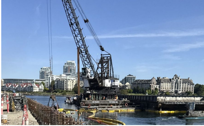
Figure 1: Progressing with installing rebar cages for the piles of the retaining wall.
