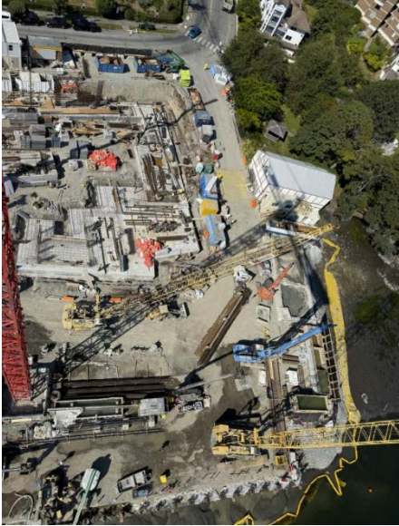
Figure 1: Progressing with the building foundation.
